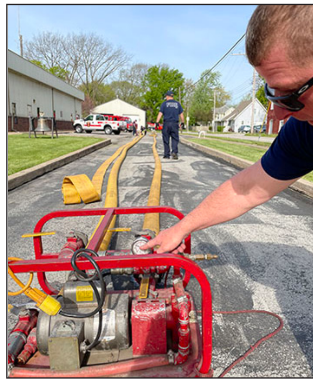
CONDUCTING AN ANNUAL TEST, Fireman Jeremy Milam points out the pressure gauge building while the fire department water hoses are attached. Fireman Jim Houk inspects the lines further down. The annual test is designed to insure the hoses will function properly under pressure when needed most: on scene at a fire.
