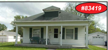
INVESTMENT OPPORTUNITY KNOCKING! Looking for the perfect investment property, look no further this 2 BR home has everything ready to go to start making income, with all appliances included. Home has a fenced in yard with a single car garage. Don't miss out call today for your private showing. $54,900 #83419
