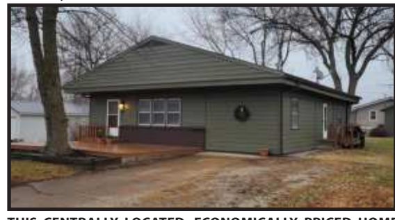
THIS CENTRALLY LOCATED, ECONOMICALLY PRICED HOME has had a total facelift inside and out! 2-BR, 1.5 BA also has a non-conforming 3rd BR or office. Original hardwood floors in the living room have been completely refurbished. Other rooms have new carpet or laminate. New paint throughout, along with new accent walls, give this house a modern feel. Nice fenced-in backyard w/ garden shed that has plenty of room for outdoor tools, or extra storage. Don't miss out on this turn-key home. $127,500 Give Hansel a call. MLS#94052
