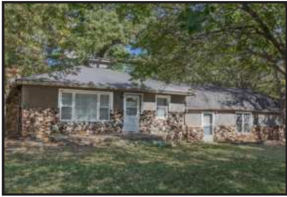
BRING THE FAMILY!! This large Truman Lake Getaway has 5BR and 3BA. Great room with cathedral ceilings, loft & wood burning fireplace, additional family/rec room with gas fireplace. Home has numerous upgrades including newer HVAC units, carpeting and bathroom fixtures. Det. 2-car garage w/loft and plenty of room for your boat & lake toys. Community boat ramp and Truman Lake just down the road. $219,900 Call Deanna for your showing today! MLS#93553
