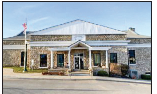
THE WARSAW CHAMBER OF COMMERCE is housed in the historic Community Building overlooking Drake Harbor.
