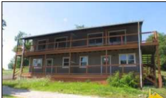
5BR, 6BA HOME W/20 ACRES +/-. Has 2-well dock w/1 lift that is included as well as 250' of seawall both w/pending permits. Excellent opportunity to build new waterfront homes. Some restrictions. Duplex on east side is finished; west side has most materials to finish. New well & State approved septic. Acreage can be excluded or divided. Call The Fannings toll free at 866-438-7070 to see MLS#79118. $259,900.
