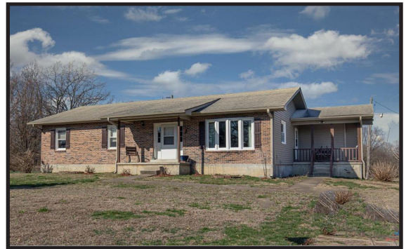
Nice hobby farm on 58 +/- acres just off blacktop road, close to town and Lake of the Ozarks/Truman Lake. 3BR home w/ full walkout basement. Also has machine shed, hay barn and several outbuildings. Storm shelter. All of this, plus much, much more. $565,000 Call Jennie for more information. MLS#94665
