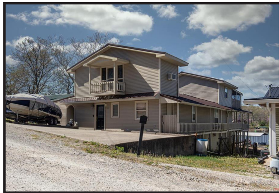
7 BR, 4 BA WATERFRONT HOME on Lake of the Ozarks. Home is in nice subdivision close to town. One-well covered dock w/ swim platform. Beautiful home on level lot. Gentle slope to water. $365,000 Call Jennie today for more information! MLS#94887
