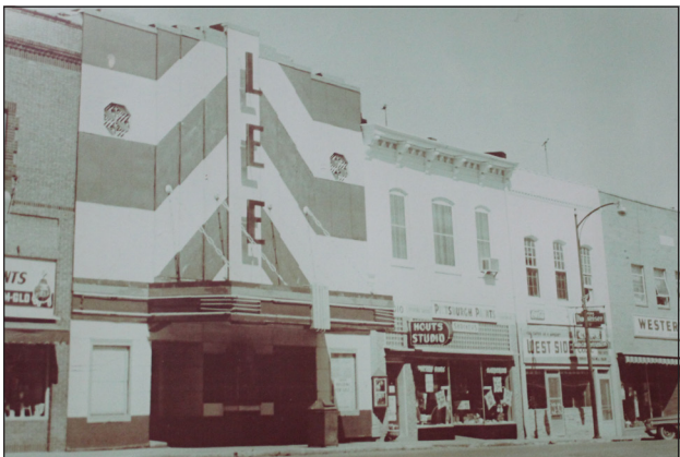
A PHOTOGRAPH of the Lee Theater, taken after an exterior facelift, which Mike thinks happened in the 1960s.
