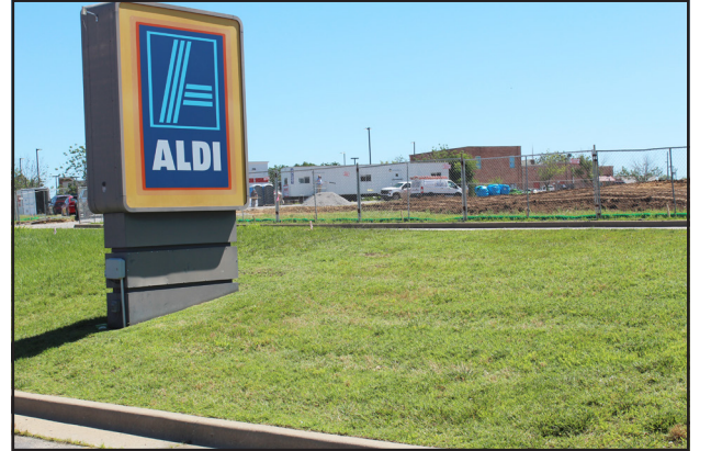
CONSTRUCTION HAS BEGUN ON ALDI'S NEW STORE.
