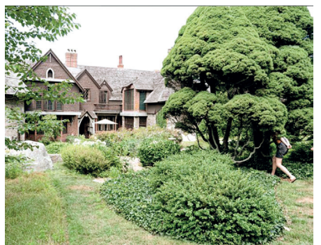
Henry Davis Sleeper House, East Gloucester
