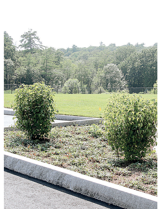
Progress continues on upper Pine Street as the "burn dump" site is converted into a much-needed sports field space.
