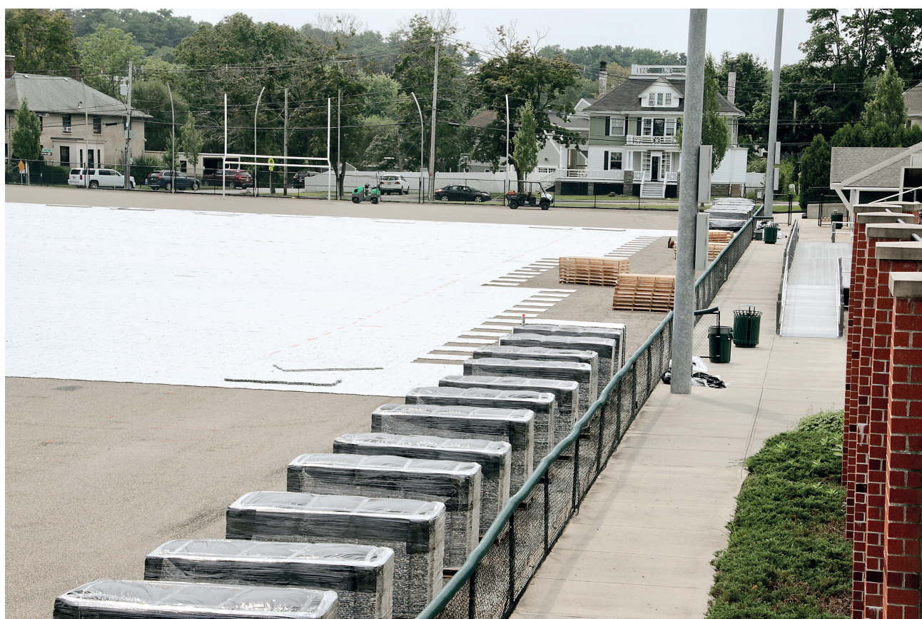
Progress continues at Hyland Field installation of new turf field.
