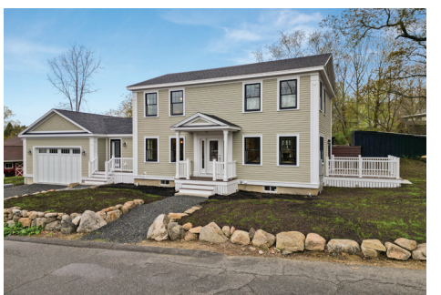
Rockport - New Construction! Beautiful colonial features an open floor plan, kitchen has 9-foot island and stainless steel appliances. $1,279,000 Kristy Aparo 978-559-1184
