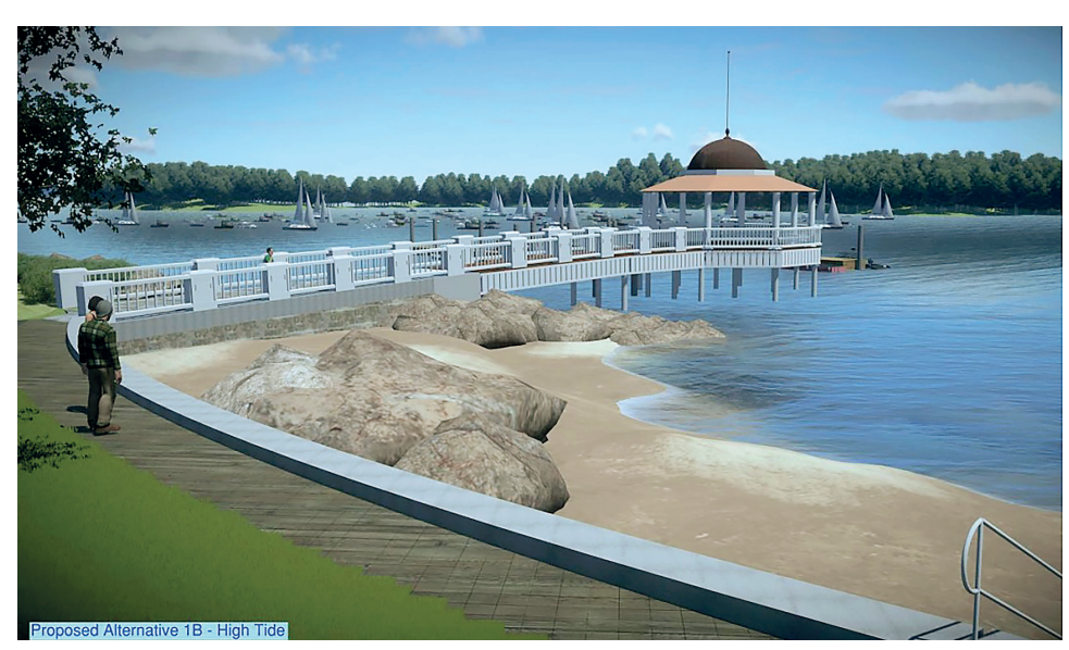
There were three options for renovating the Rotunda to meet new federal standards for tide surges, but in the end the Select Board voted for Option 1, seen here, in which encased steel pilings would raise the structure to 19' on its current footprint, costing $2.3 million. (Image: Foth Engineering 2023)
