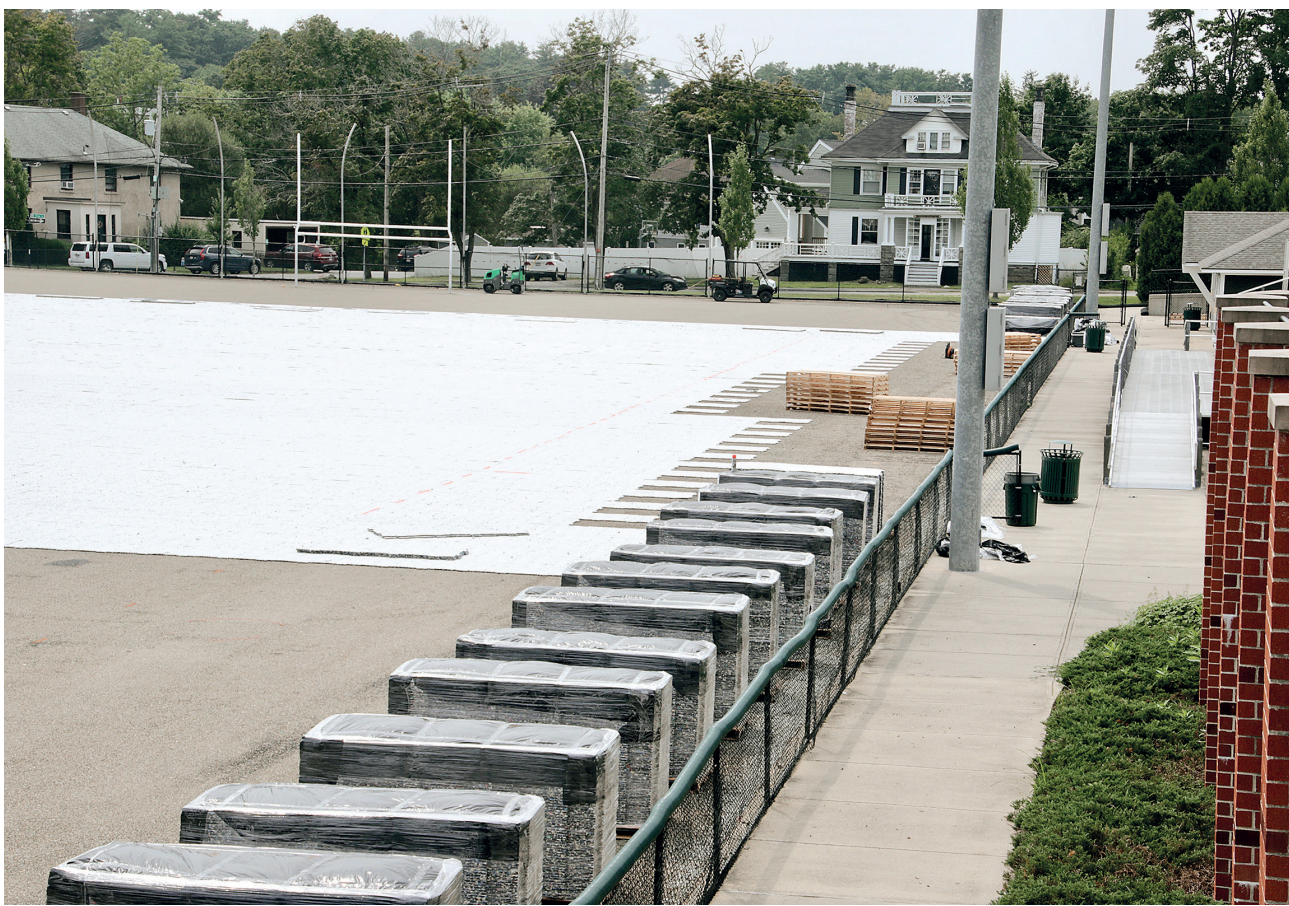
Progress continues at Hyland Field installation of new turf field.
