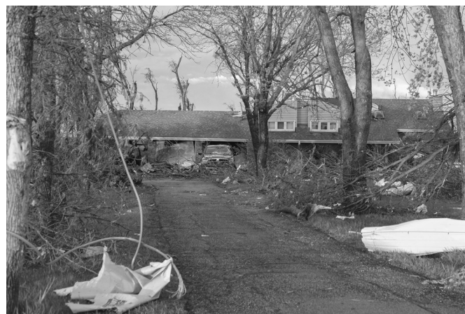
JOE BURNS | OAKLAND INDEPENDENT A severely damaged home along Highway 133 at Todd Drive.
