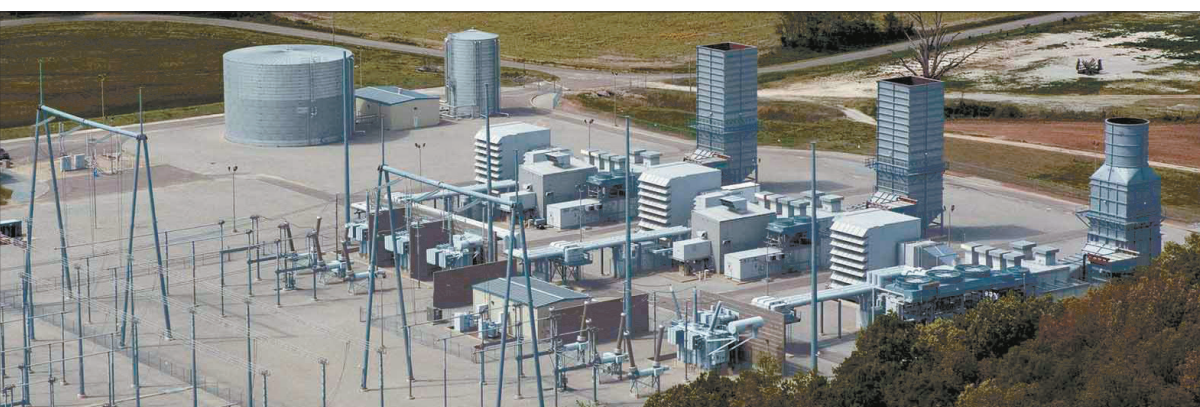
The Gleason Combustion Turbine site sits on 97 acres in Weakley County, Tenn. in Gleason and is visible from State Route 22. The plant consists of three simple-cycle Siemens-Westinghouse combustion turbines. The three combustion turbines have a combined generation capacity of 500 MW. TVA is considering a proposal to upgrade the site to a combined-cycle plant, which would add an additional 350 MW of capacity.
