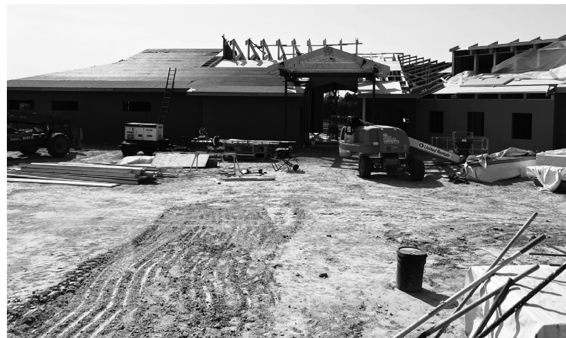
The Willow Lake Nature Center is expected to open in the spring of 2023. Construction on the building started roughly one year ago.
