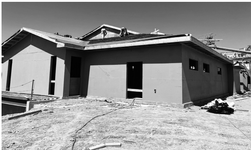
PHOTOS COURTESY OF SCOTT NELSON Roofing is installed at the Willow Lake Nature Center.
