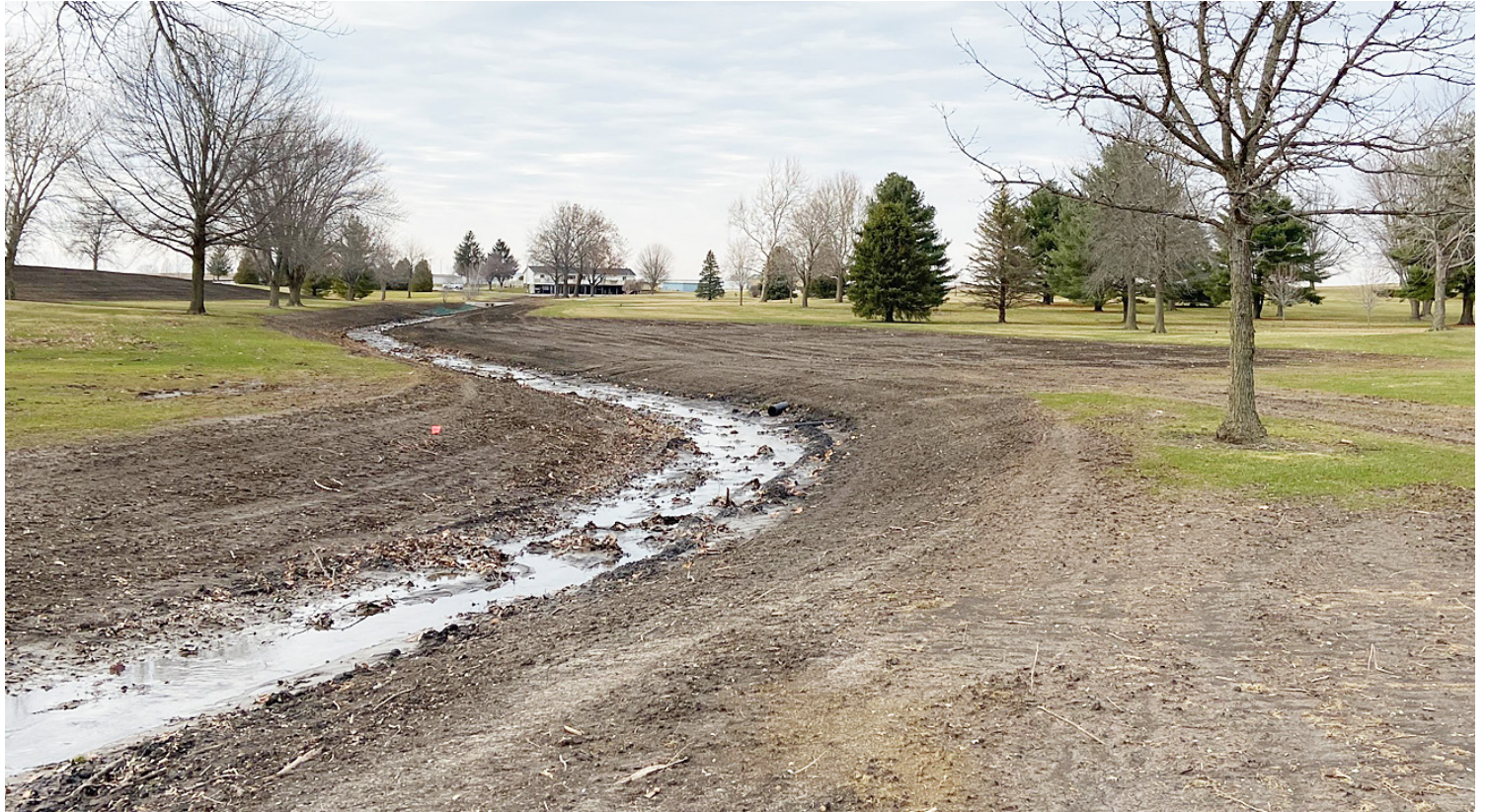
Wahkonsa Country Club has added a man-made creek along hole No. 7 to help with continued water drainage issues. Needham Excavating of Walcott helped shape the new feature, which will direct water from the course along hole No. 7, south through holes 8 and 5 toward Highway 6. Photo by Derek Sawvell
