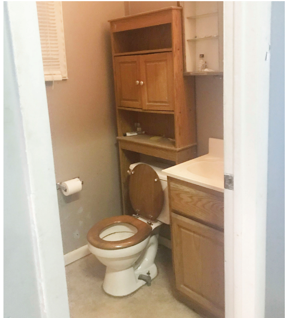
This 100-year-old property was previously a duplex rental, complete with one bathroom on each floor. The upstairs bathroom received a new tub/shower, toilet, a maple double vanity and linen cabinet.
