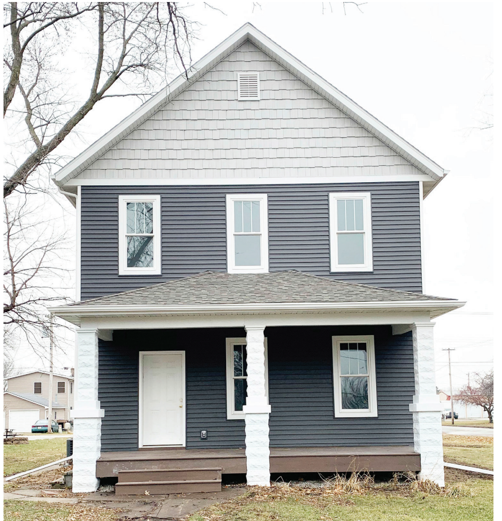
The house above in Durant was built over 100 years ago and is located at 1101 Sixth Street. Originally built for a single family, the house had previously been transformed into a duplex rental for many years. After purchasing the house in 2015, Paper's Construction Company had visions of remodeling the house and restoring it back to a single-family dwelling, which began in late 2018.
