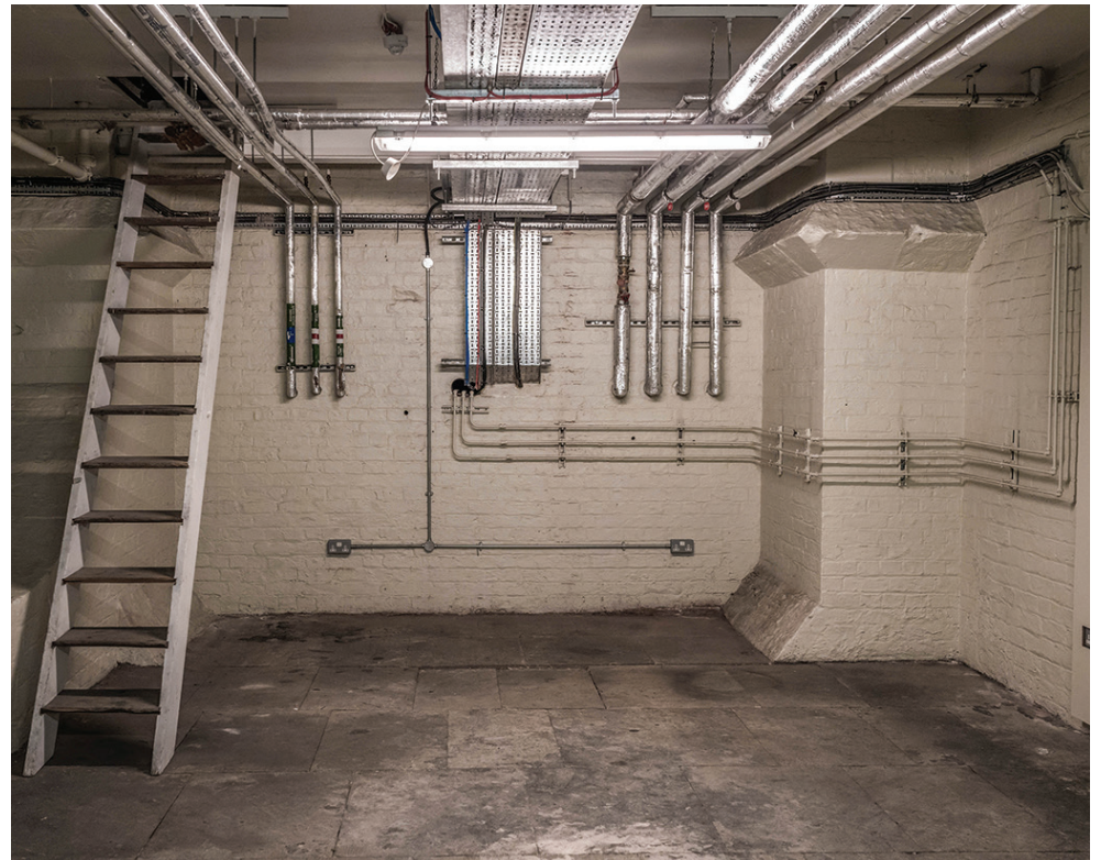
Remediating water issues in a home generally breaks down into two methodologies: exterior waterproofing and interior waterproofing.
