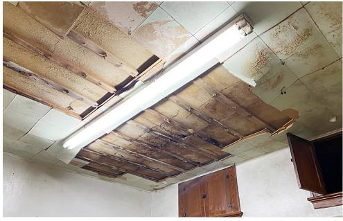
Roofs on both of the Legion buildings along Fifth Street in Durant are in a state of disrepair, resulting in water damage to the interior ceilings of both structures, as shown in the photo above. After planned renovations, the two structures will be mated into one large frontage under one roof. More photos and the building plans are available online at wdadvocatenews.com.
