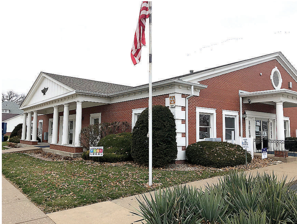
US Bank will vacate the attractive colonial-style professional building in downtown Eldridge effective Jan. 2, 2021.
