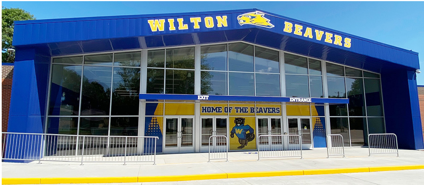
The exterior to the new Townsend Commons at Wilton High School is pictured above. The commons is attached to the south end of the high school gym, and features a new concession area, commons, restrooms, office space, TVs, ample seating, and eventually more furniture and trophy cases. Photo by Derek Sawvell
