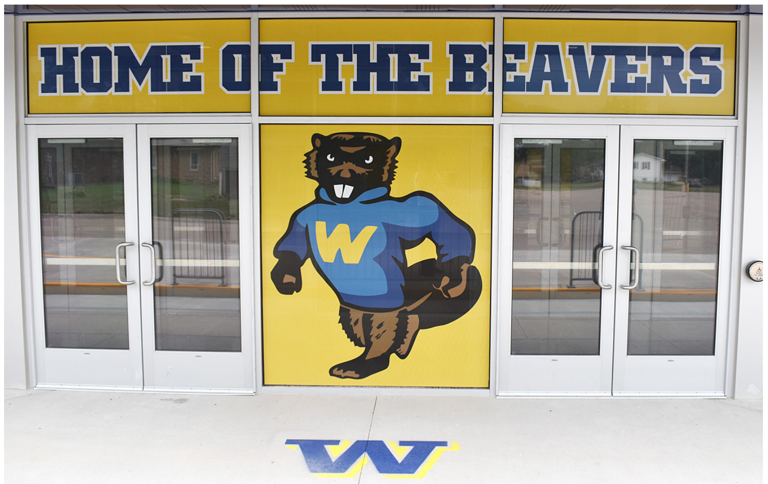
The entrance to the Townsend Commons is pictured, with fresh school logos and the message, "Home of the Beavers." An old vintage Beaver logo was placed between two sets of double doors that will take students and visitors into the new commons on the south end of the high school gym. Photo by Derek Sawvell
