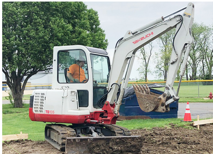
Durant High School's ACE Mentoring program was fortunate to have some grants and donations in order to purchase a mini excavator (pictured) from Star Equipment.
