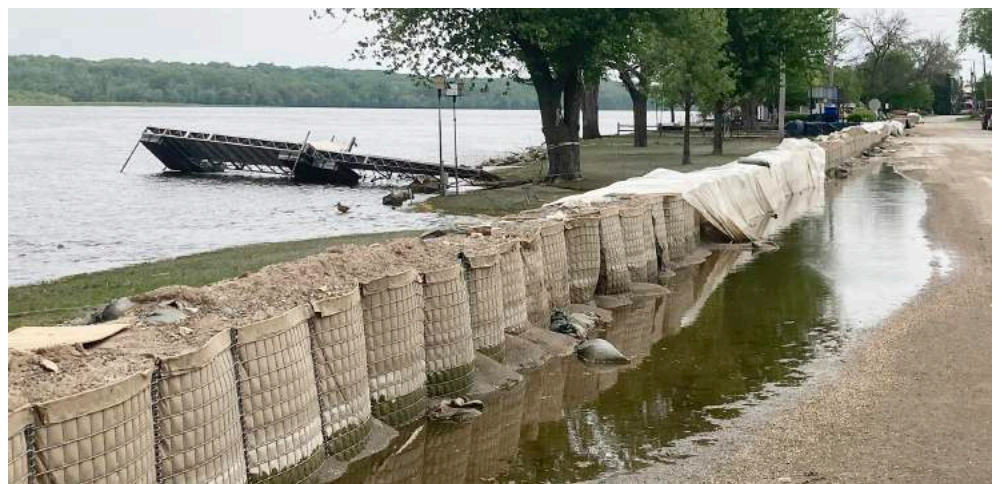
Princeton's quarter-mile of floodwall awaits dismantling.
