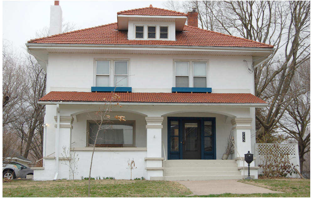
715 N. Calhoun used to be a nursing home and now houses a family.
