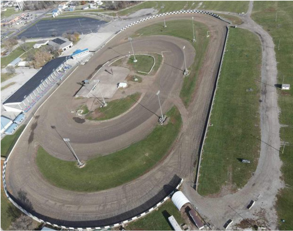
The quarter-mile track within the half-miler is being lengthened for a longer front straight, more wedge-banking, and less of a bowl.
