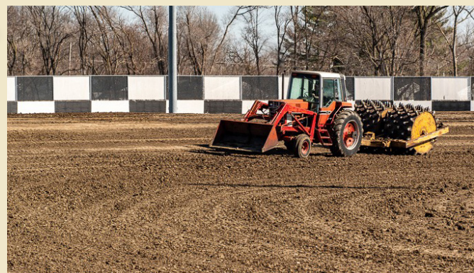
Struck grades track banking in preparation for the season.
