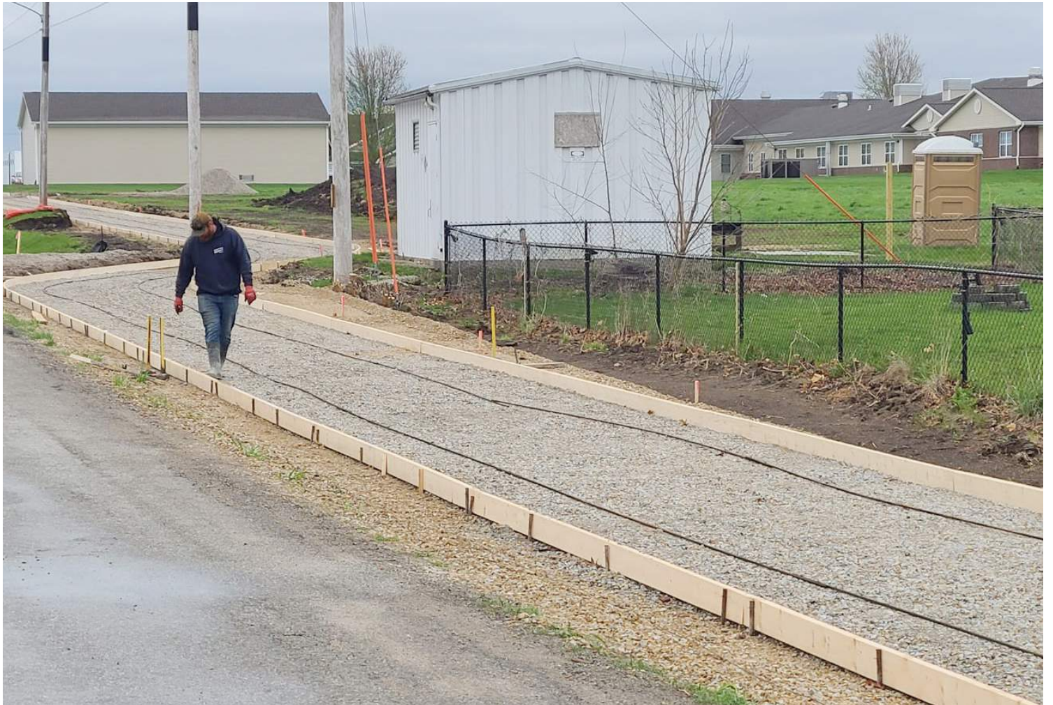
Hoekstra Masonry crew member checks framing on a sidewalk the company built in Wilton last week.
