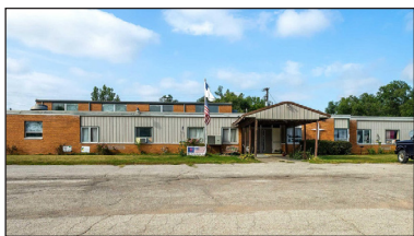
1951 Yellow Ave, Montpelier--Versatile commercial property with ENDLESS possibilities. 11,771 SF main building, with attached 2,904 SF gymnasium. All sitting on just over 8 acres!
