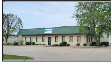
502 Ayres Progress Dr, Wilton--Commercial/Industrial steel framed structure w/100x120 warehouse w/18' sidewalls & radiant heat, loading dock, overhead door, 2 electrical services.
