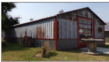
112 Main St, Bennett--Steel building currently operating as Ol' Biggs bar & special events center. New concrete patio, which is covered. Concrete bar, 2 bathrooms, and stage.
