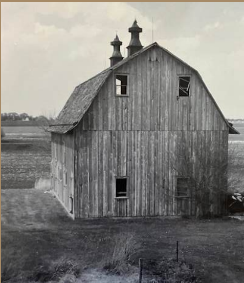
Barn on the Arp farm south of Eldridge.
