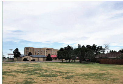
E. 28th Ave. Pampa Commercial Lots
