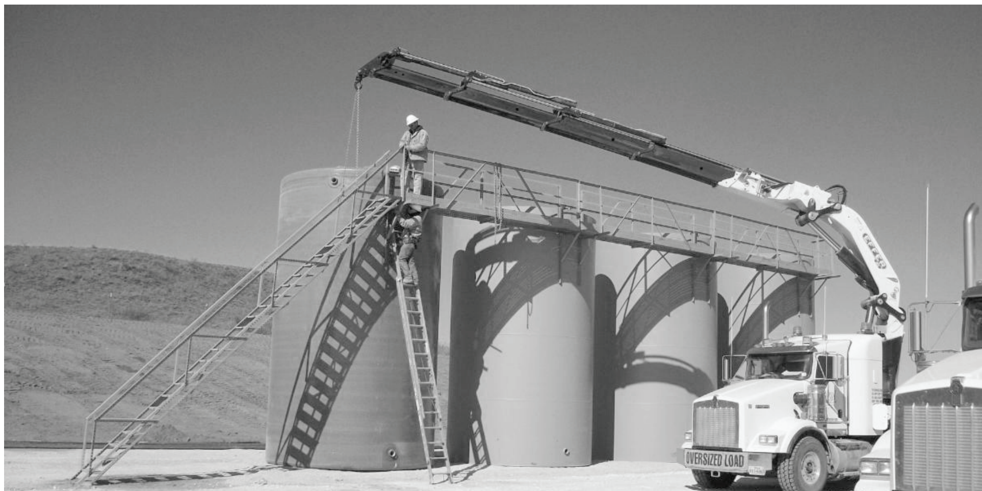
WW Employees on job Site
