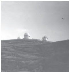
VIEW FROM BELOW — About midway through the valley the site appears in profile on the mountain top. (This was taken with a telephoto lense.)
