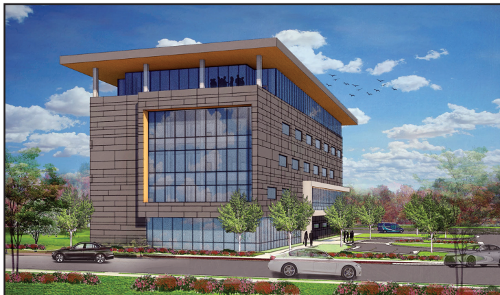
Cone Health will open urgent care and primary care medical offices on the first two floors of the four story, approximately 54,000 sq. ft. building. The health care provider expects 25,000 people a year to use those facilities.
