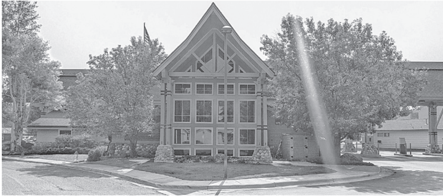
Sometime between the afternoon of Aug. 21 and the morning of Aug. 23, someone apparently used a BB gun or similar weapon to shoot some of the large windows at First Bank of Wyoming in Cody. The damaged windows were located at the very top of the tall building and face west, say Cody police, who believe the windows were shot from the area of Platinum Avenue. Anyone with information about the incident is asked to contact Cody Police Sgt. Beau Egger at 307-527-8700 or to submit an anonymous tip at www.bit.ly/3DxYixW . Photo courtesy Cody Police Department
