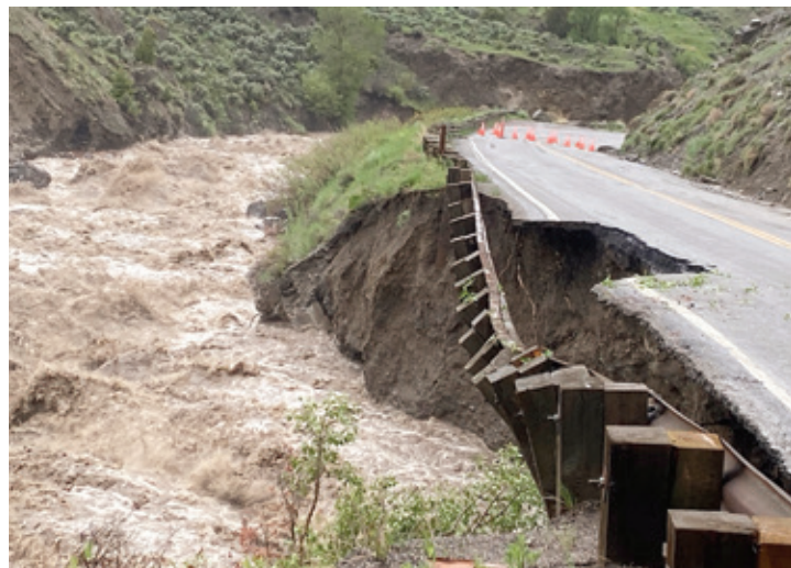
A section of road near Mammoth Hot Springs, in Yellowstone National Park, washed away Monday. Much of the road through Gardiner Canyon near the park's North Entrance has washed away, including the Carbella Bridge, in Gardiner. Photo courtesy of NPS
