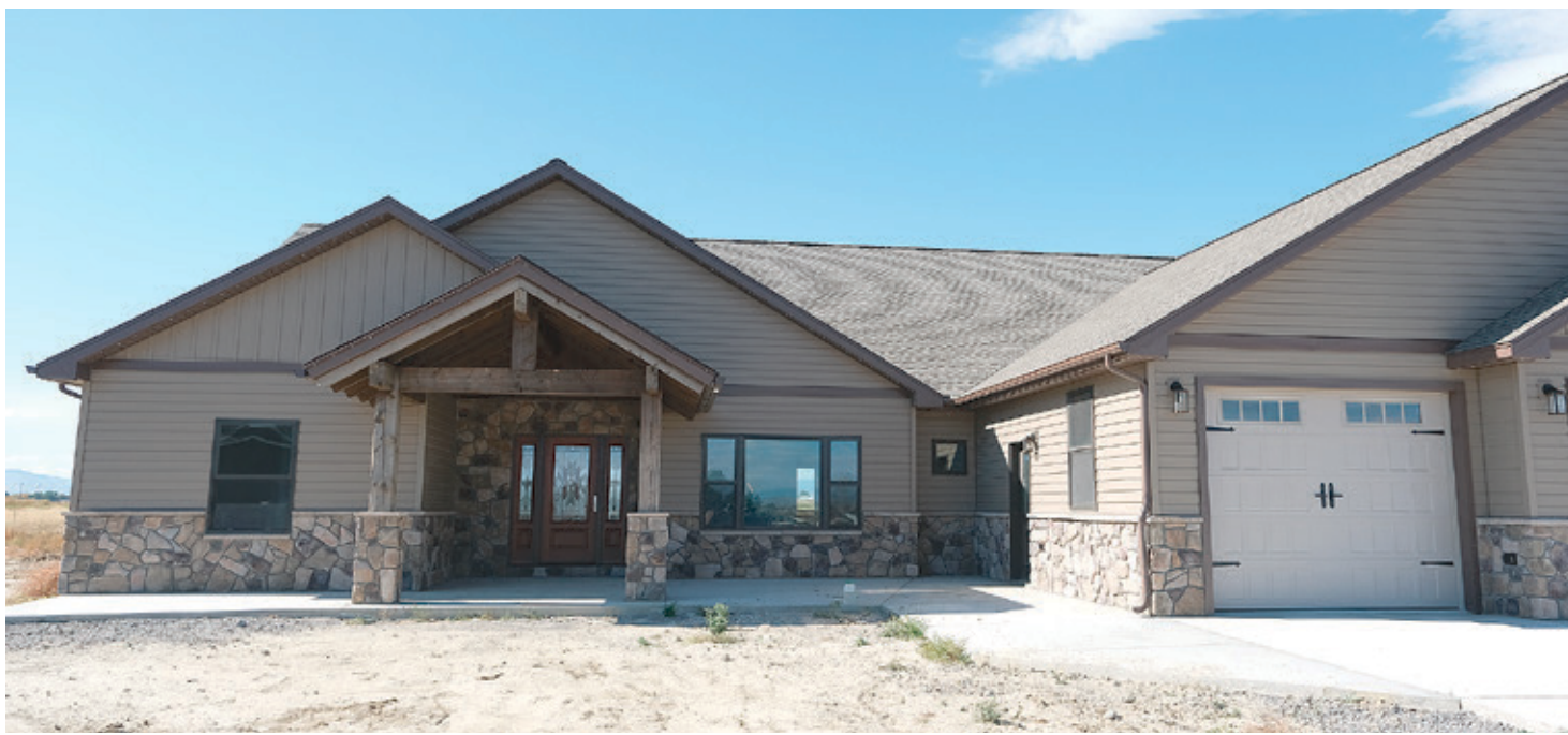
Metzler Construction is nearing completion on Mike and Kay Regan's 3,500-square-foot home at Campfire Lane. Having a view of Heart Mountain was a priority of the well structured house. Tribune photos by Braden Schiller
