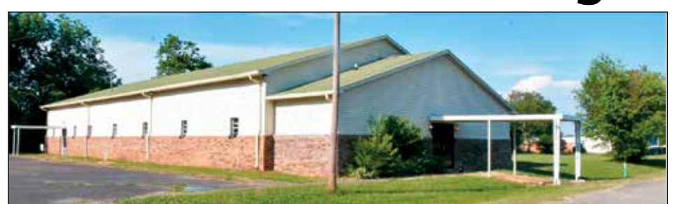
OBION RIVER ASSOCIATION HEADQUARTERS - The Association, composed of Missionary Baptist churches from 9 surrounding counties, was heavily damaged by second act of vandalism.
