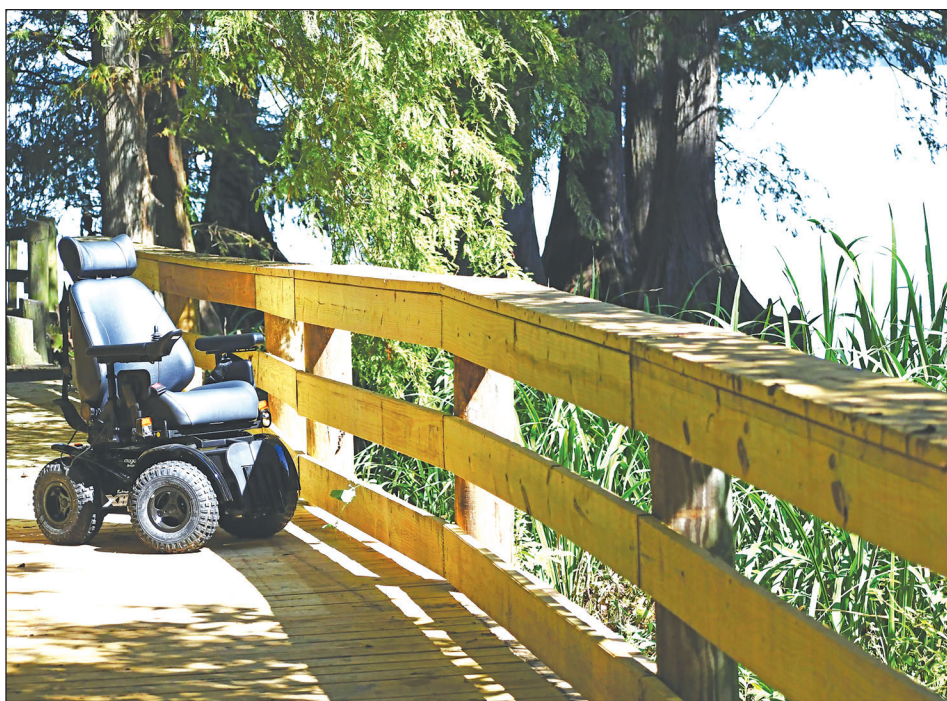
REELFOOT LAKE PIERS MADE HANDICAP ACCESSIBLE - Reelfoot Lake State Park recently announced that several of the public access piers and walks at the park have been made wheelchair accessible. Also several of the walkways and piers have recently been rebuilt and repaired - Submitted photo
