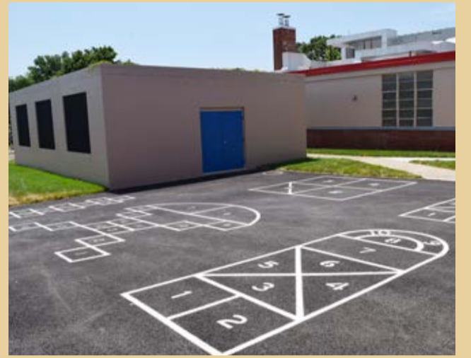
Riviera Beach Elementary will unveil its new early childhood education wing for the 2019-2020 school year after more than one year of construction.
