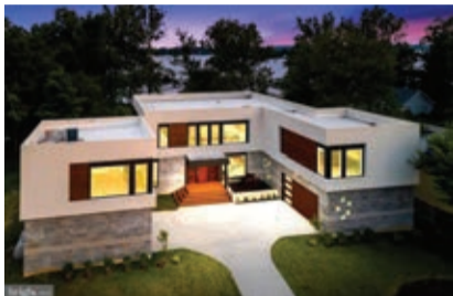
Custom-Built Waterview Home 328 Hickory Point Rd, Pasadena - $1,495,900
