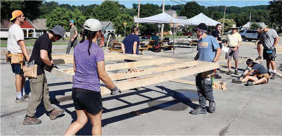
The WoodsWork team constructed walls in an offsite parking lot before taking them back to the house. WoodsWork's manpower shaves months off the time it would take Habitat for Humanity to complete a home.
