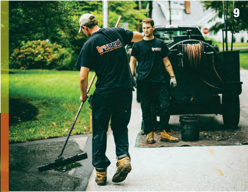
Ian Chaput TruSeal Asphalt and Concrete
