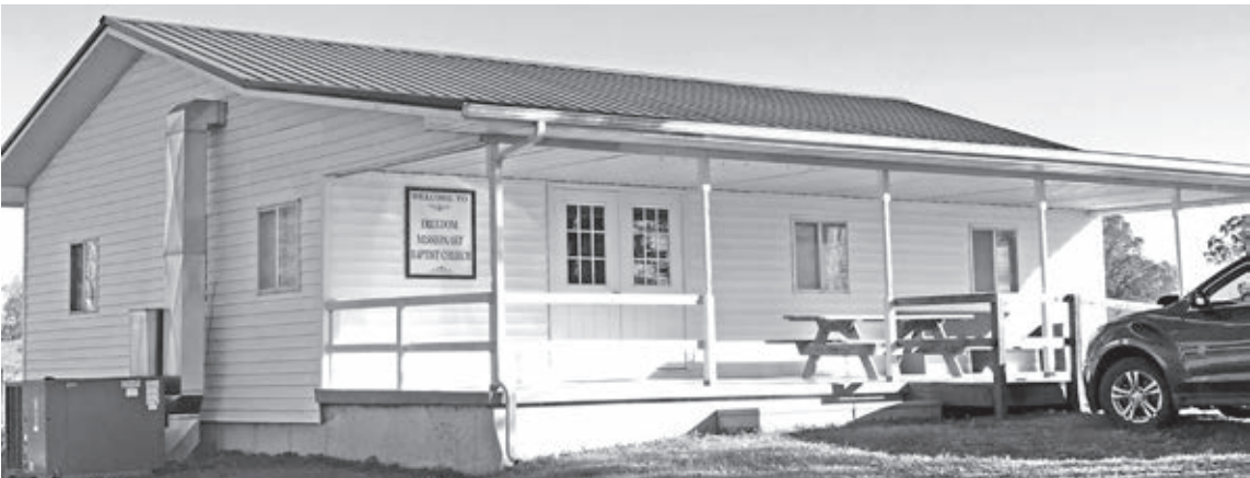
FREEDOM MISSIONARY BAPTIST CHURCH North Street out of Stockton 5 miles to E. 932 Road
